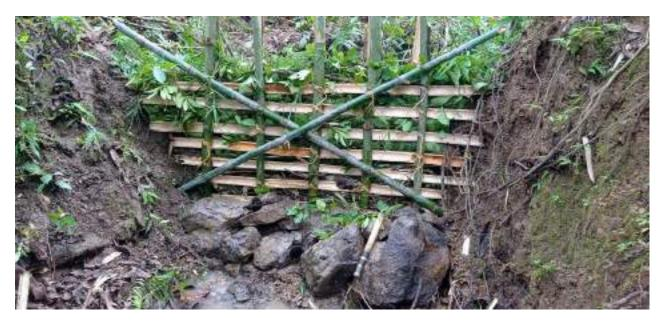
Brushwood check dams are made of posts and brush are places across the gully. The main objective of Brush wood Dam is to hold fine materiel carried by flowing water in the gully. Small gully heads, no deeper than one meter, can also be stabilized by brushwood check dams.
